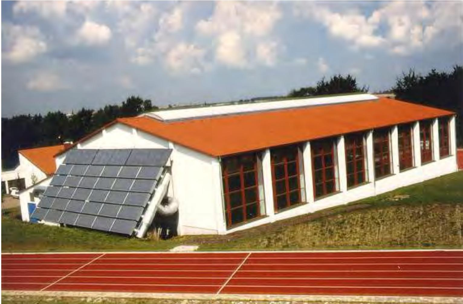
75 m<sup>2</sup> GLK, 50° Fassade, Luftmenge max. 8.000 m<sup>3</sup>/h, 45 kW<sub>p,therm</sub>.
